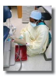
Photograph showing the used filter disconnected from the vacuum lines. The red vinyl caps are securely placed on both ends and the used filter is ready for recycling. A new DD2011 amalgam separator can now be installed by placing the vacuum hoses on the appropriate hose barb fittings.
